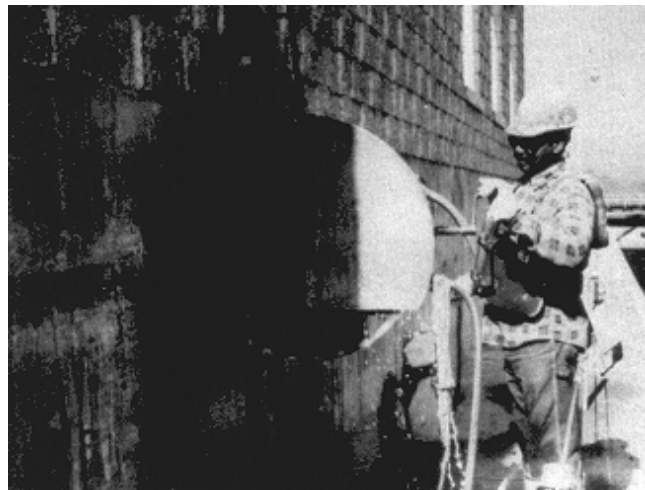
Figure 5-3. Diamond-blade saw
