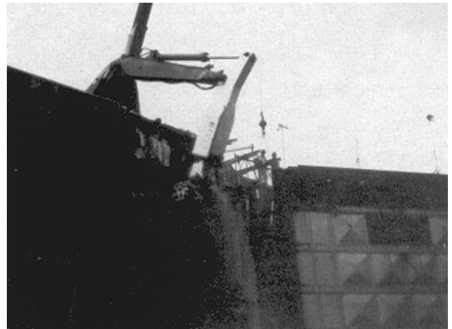
Figure 5-11. Rotary-head milling
