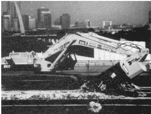
Figure 5-2. Boom-mounted concrete crusher
